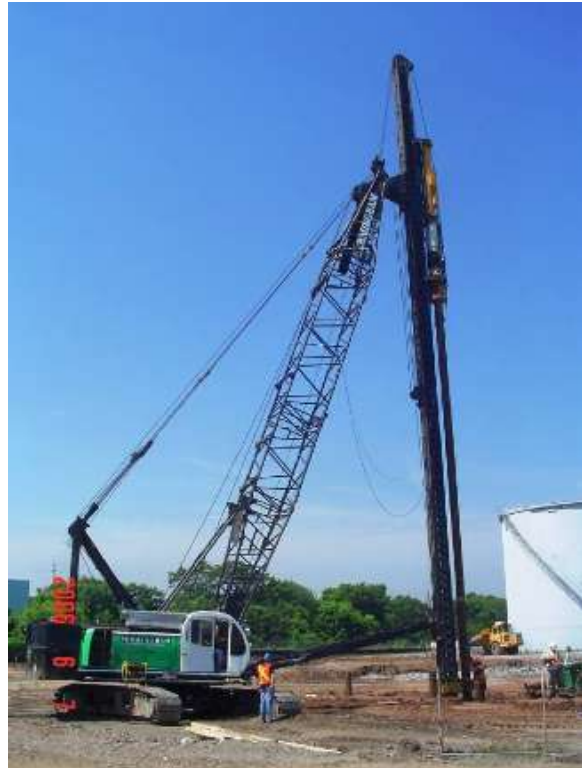
Figure 17 – Crane, fixed-lead and Diesel Hammer
