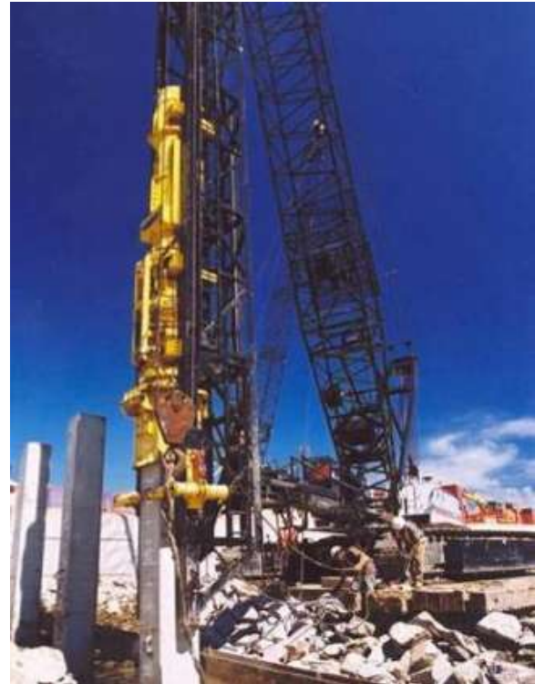
Figure 10 – B-6505 Hammer driving 24-in concrete piles at the Woodrow Wilson Bridge
