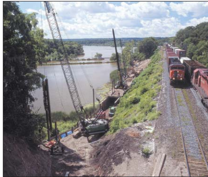
The constructed trestle became part of the permanent wall.
