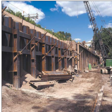
Transition from tie-back wall to self-supporting wall.
